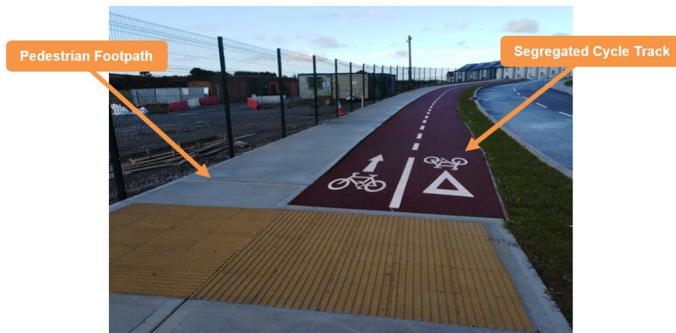
Figure 11.11: Pedestrian and Cycling Facilities At Ballygossan Park Site Access
